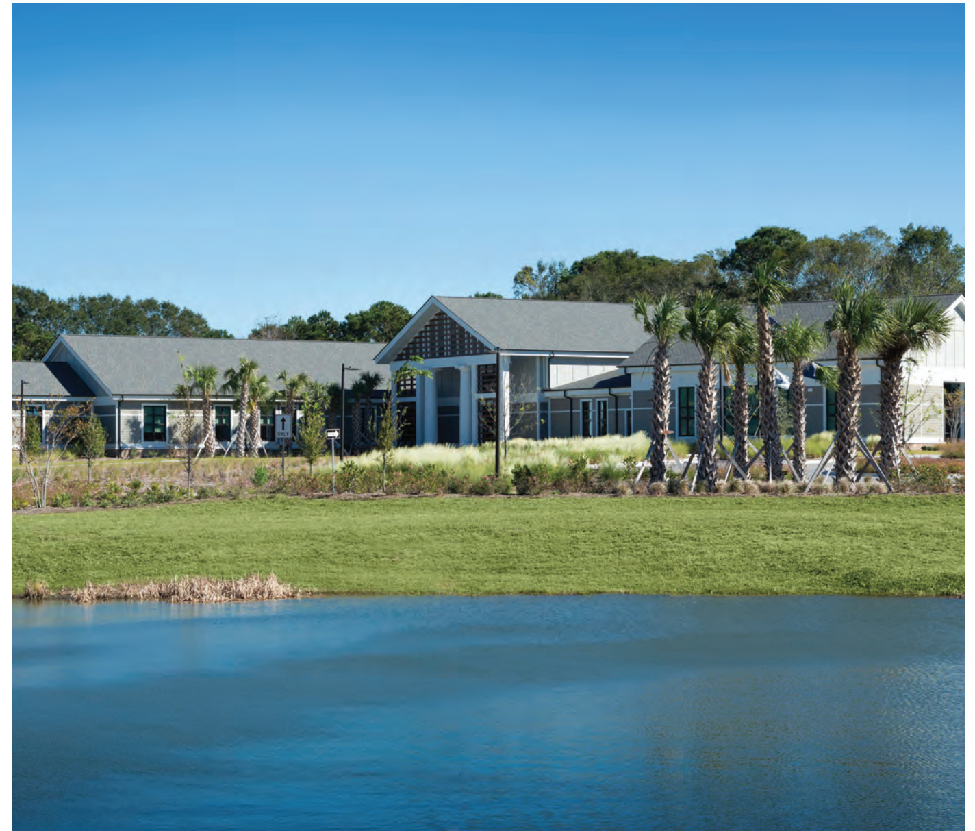
The Town's Municipal Center Complex
